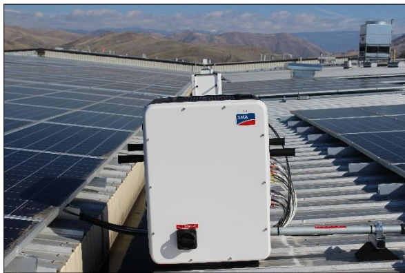
Pickett Solar uses SMA CORE1 inverters for a commercial installation in Sanger, Calif.
